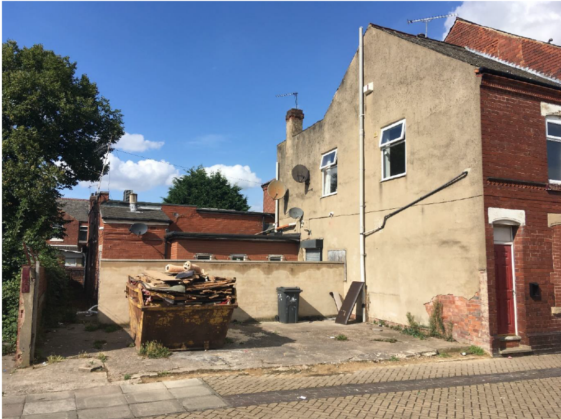
Photo 3 – Application Site: rear yard, including parking area (for flats above) and access for deliveries
