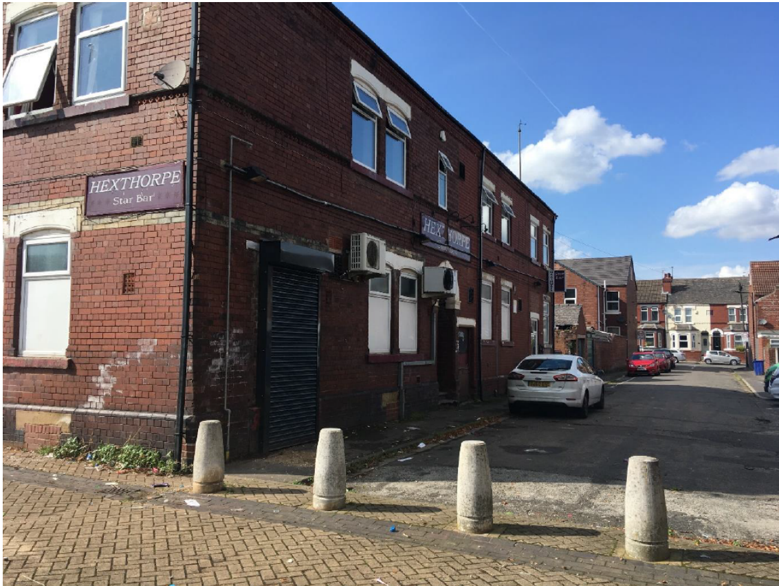
Photo 1: Application Site: Elevation at Langer Street
